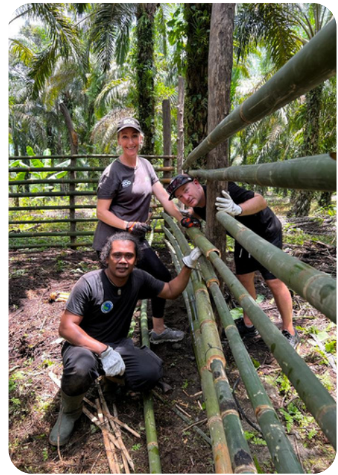
Livestock corral construction
