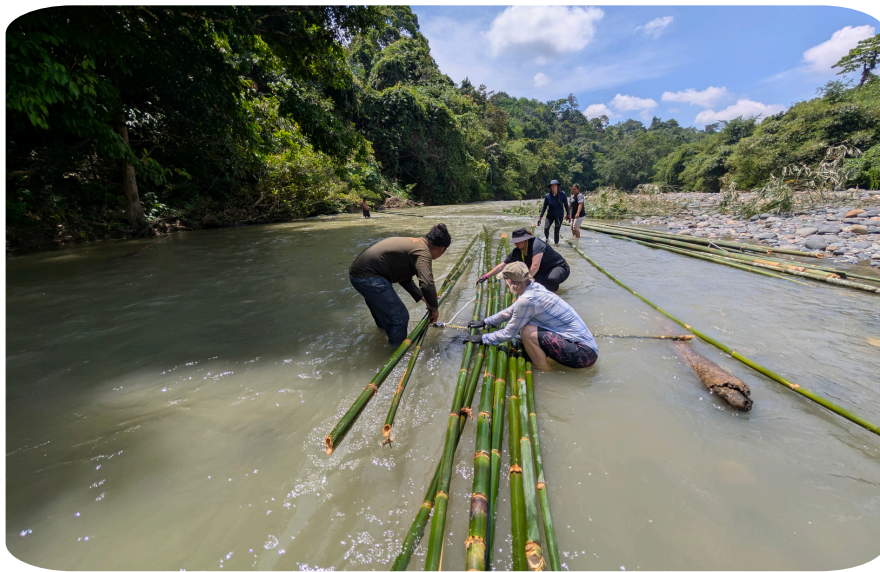
Constructing the livestock corral
