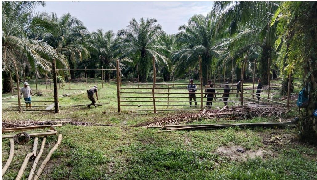
Construction of corral 13
